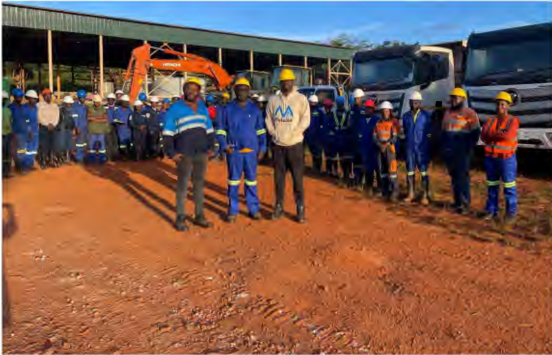
Figure 7: Metalex team at work at the Project Site
