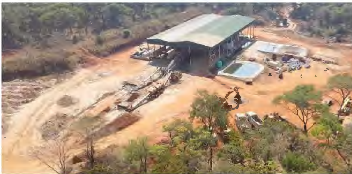
Figure 2: Existing Processing Plant
