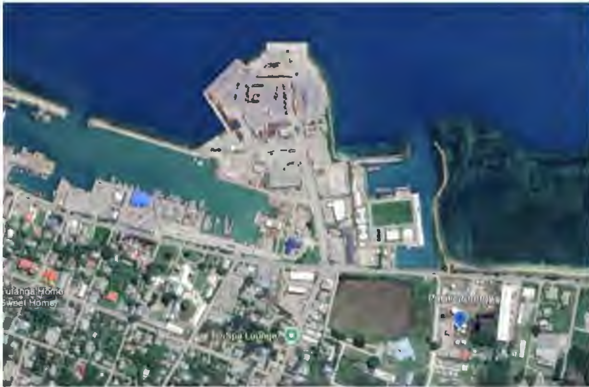
Figure 3 – Touliki Wharf Area
